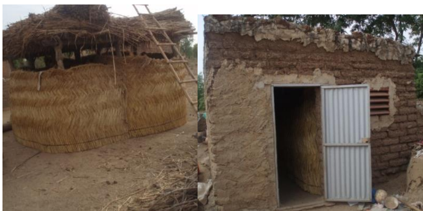
Figure 1: Overview of the type of village chickens housing used for the experiment
