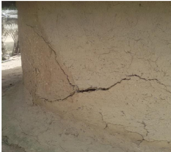
Plate 2: A cracked house and a collapsed house caused by flood in Lau 1
