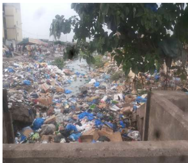
Photo 6: Clogged outlet in the Divo II district
